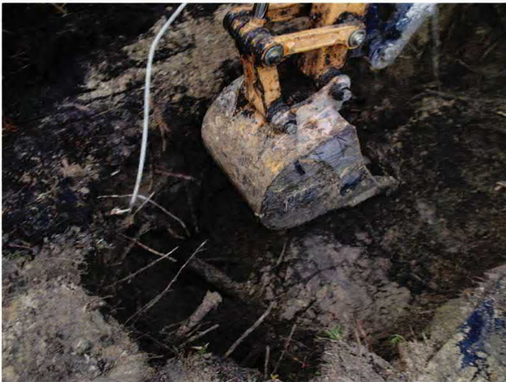
Picture 2: UST 560Dahlia removal in progress.
